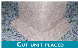
CUT UNIT PLACED
