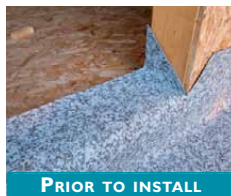
PRIOR TO INSTALL
