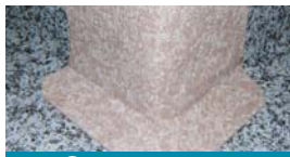
CUT UNIT PLACED
